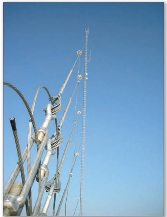
Two PRPC-owned towers were purchased this past year, saving $36,000 in annual lease expenses.
